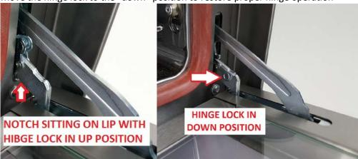
3. Do NOT leave the Hinge lock in the "UP" position at the end of installation
